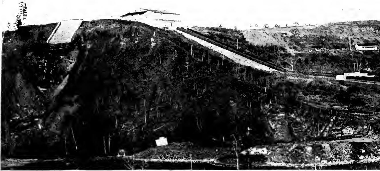
General View of the Kaministiquia Power Company's Hydro-electric Station at Kakabeka Falls—Shows Forebay and Spillway
